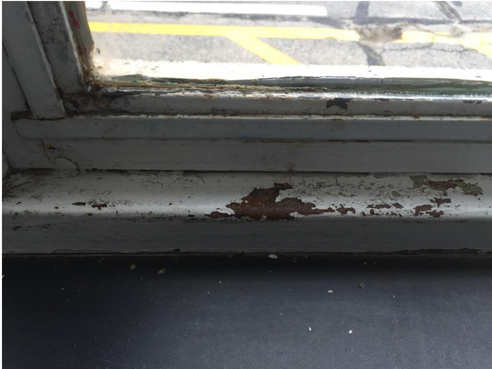
South School Window Replacement
